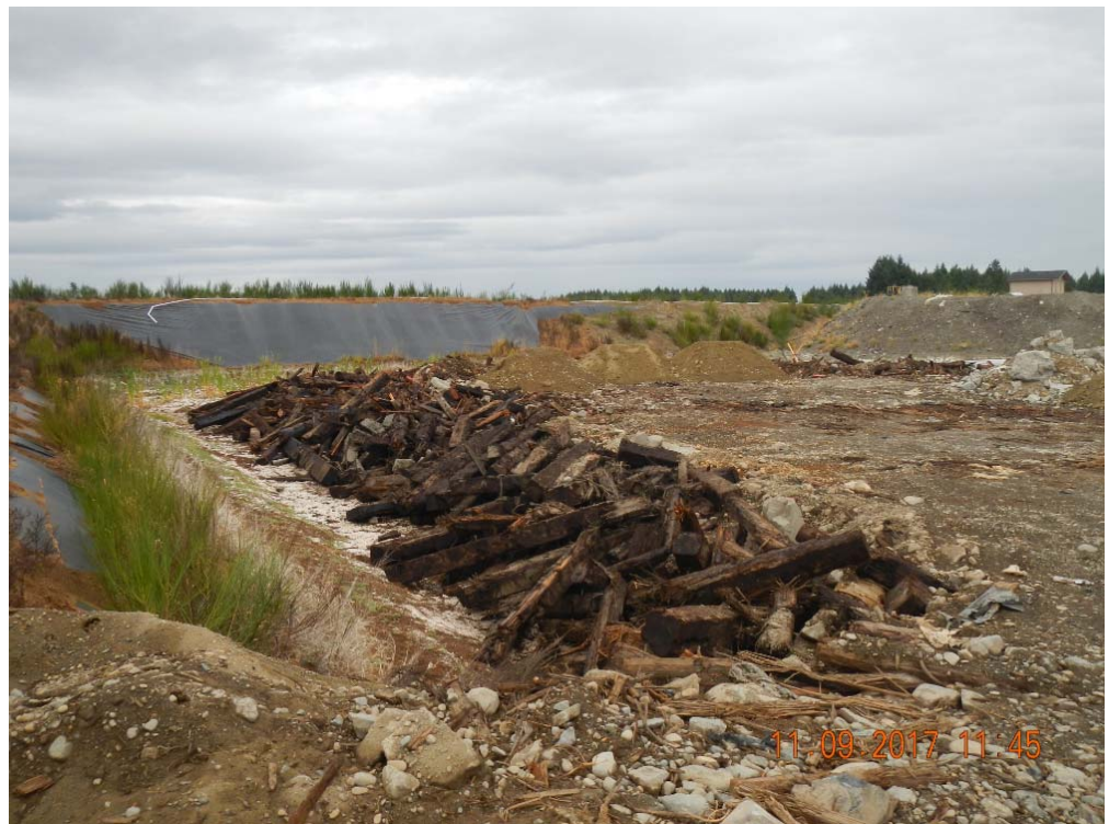
Photo 1 Lined landfill area with creosote logs.
